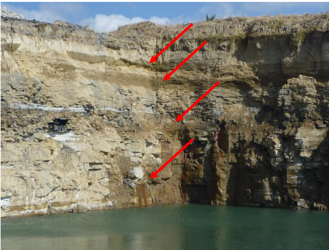
Figure 22 Opencast mine profile indicating numerous distinct flow paths (arrows) through the exposed profile (soil, weathered sandstone, carbonaceous shale, hard sandstone)
