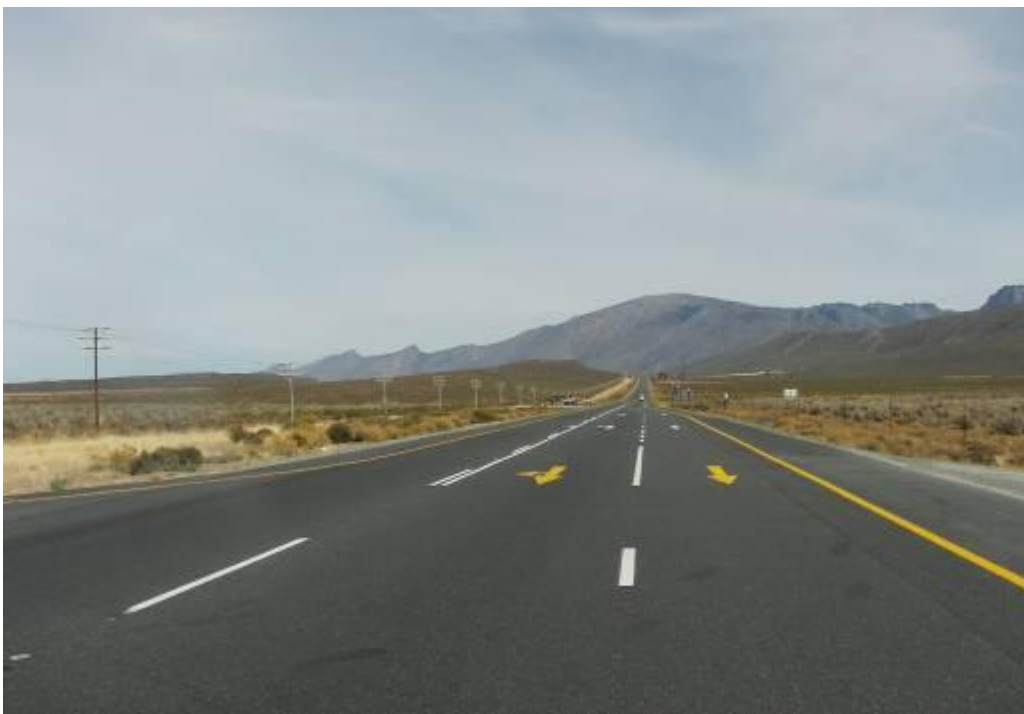
Road conditions on top of the Hex River Pass
