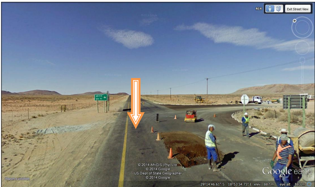
Figure 2-3: Proposed access point to Namies Suid/ Poortjies site adjacent to N14 – street view
