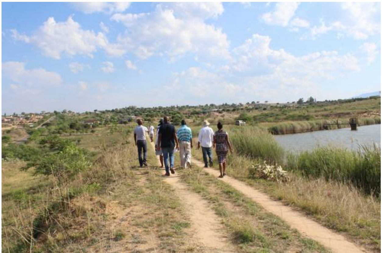
Figure 3: Delegates inspecting the Casteel Dam embankment heading towards the intake tower.
