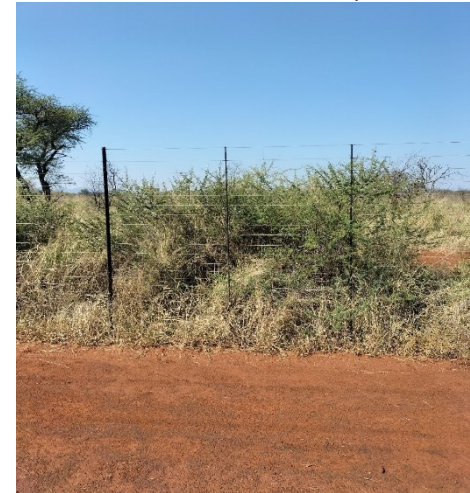
Figure 30: Nyala 2 SEF South East Corner – South West View (GPS 24°56'3.53"S 27°19'6.81"E)
