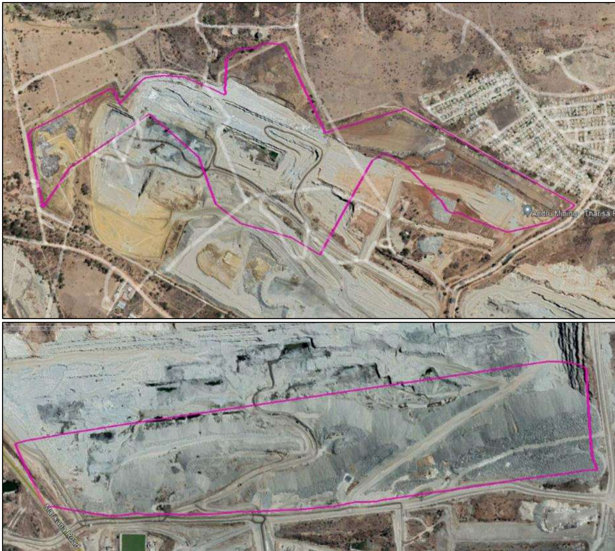
Figure 2: Images illustrating the extent of transformation within the West Above Ground WRD (top image) and the East Above Ground WRD (bottom image). From the images, it is evident that vegetation is largely lacking, especially within the pits. Surrounding vegetation (i.e., around the pits) is lacking because of historic clearing and mining activities. Google imagery as of June 2022.
