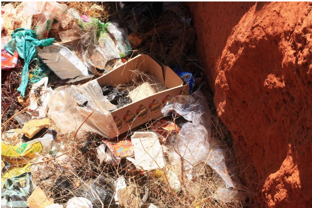
Photo 4 Rubble that gathered at eroded area at the site. Photo: R.F. Terblanche
