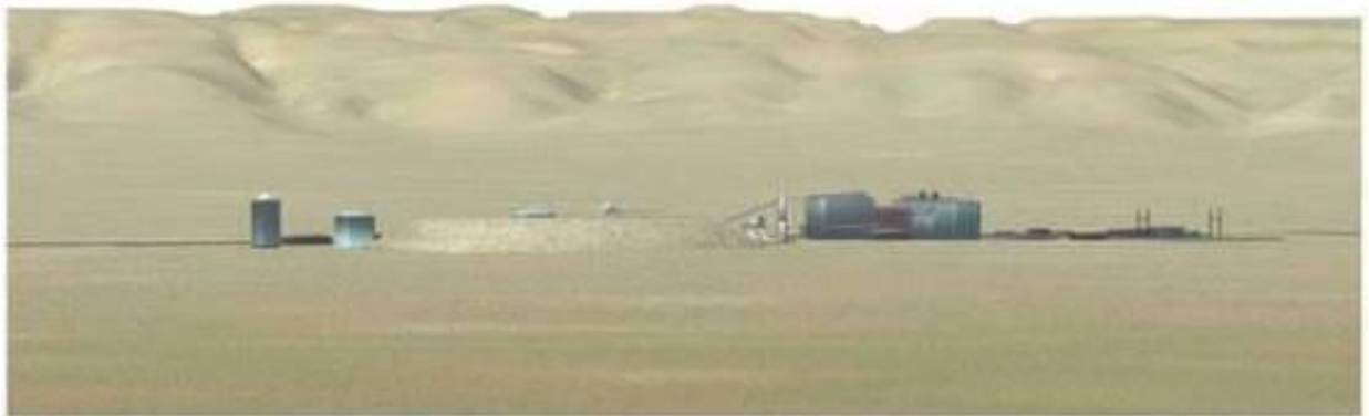
View from 3 000 metres
