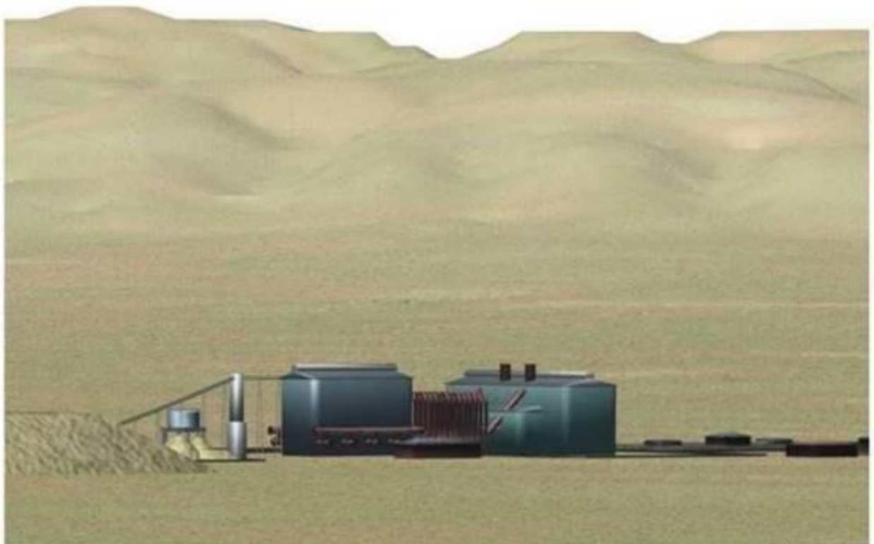
View from 1 000 metres
