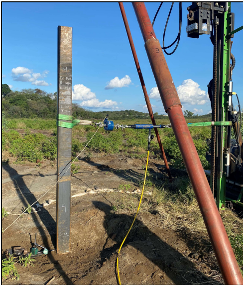
Figure 6: Lateral load test setup 1
