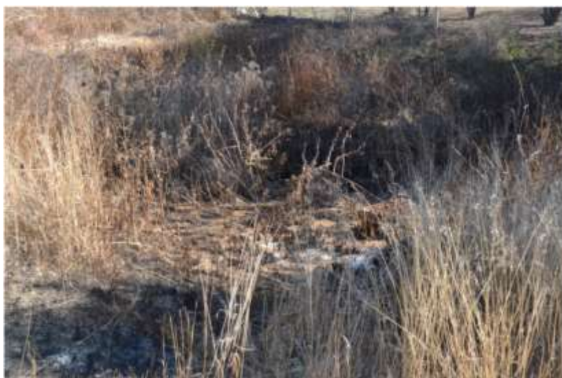
Figure 10: Sludge drying bed
