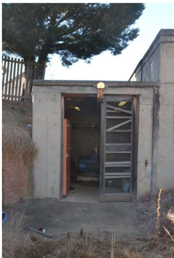
Figure 12: External view of clearwater pump station
