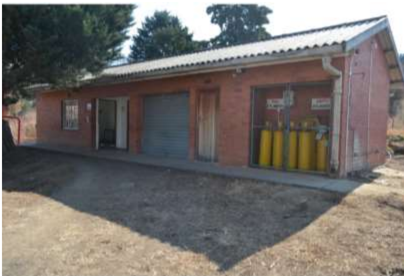
Figure 15: Existing treatment works building
