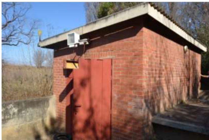
Figure 1: External view of raw water pump station
