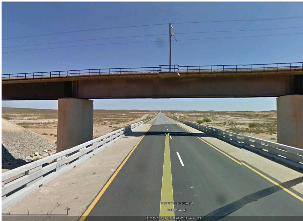
Overhead Railway Bridge on N7, Vanrhynsdorp
