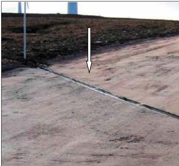
Figure 2-3: Cross drains under the Internal Roads
