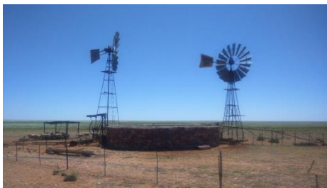
Plate 4 – Windmill-driven boreholes and reservoir
