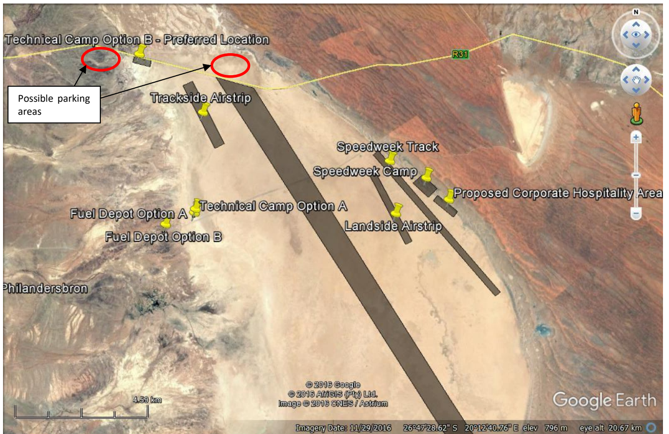
Figure 1: Google Earth image showing the various infrastructure and components of the Bloodhound SSC project (including the various options/alternatives) at Hakskeen Pan.
