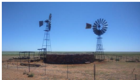
Plate 4 – Windmill-driven boreholes and reservoir
