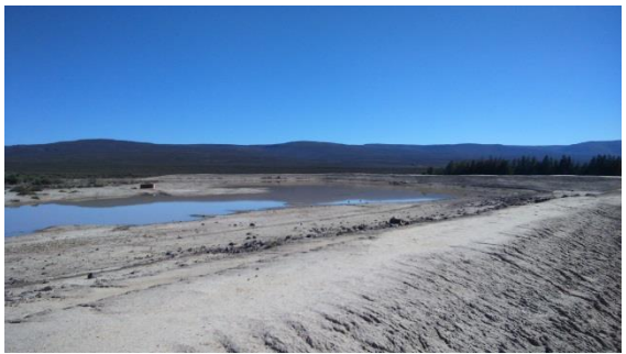
Plate 6: Earth-wall dam with water
