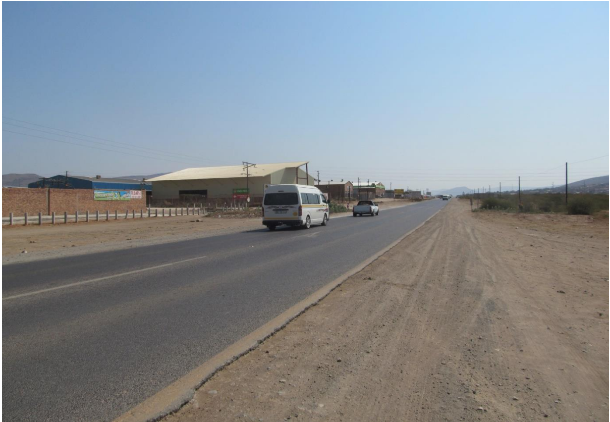
Photo 15: At km 142 to the North West
