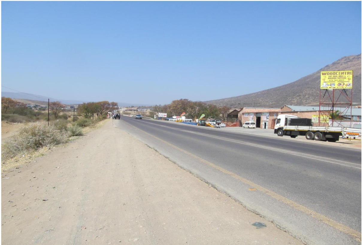
Photo: At km 142 to the South West
