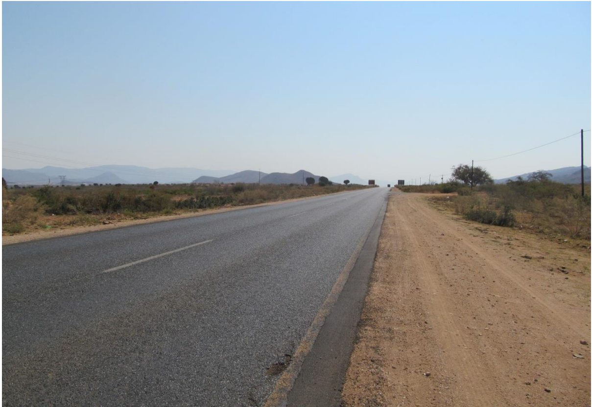
Photo 5: At km 117 to the North West
