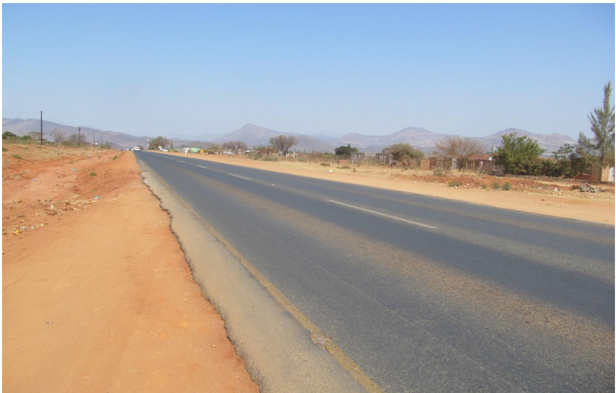
Photo 10: At km 127 to the South West
