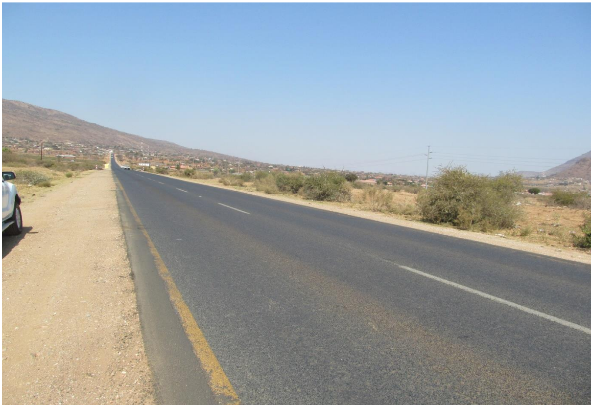
Photo 6: At km 117 to the South West
