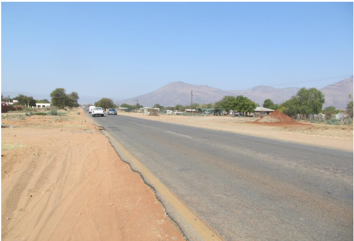
Photo 14: At km 137 to the South West
