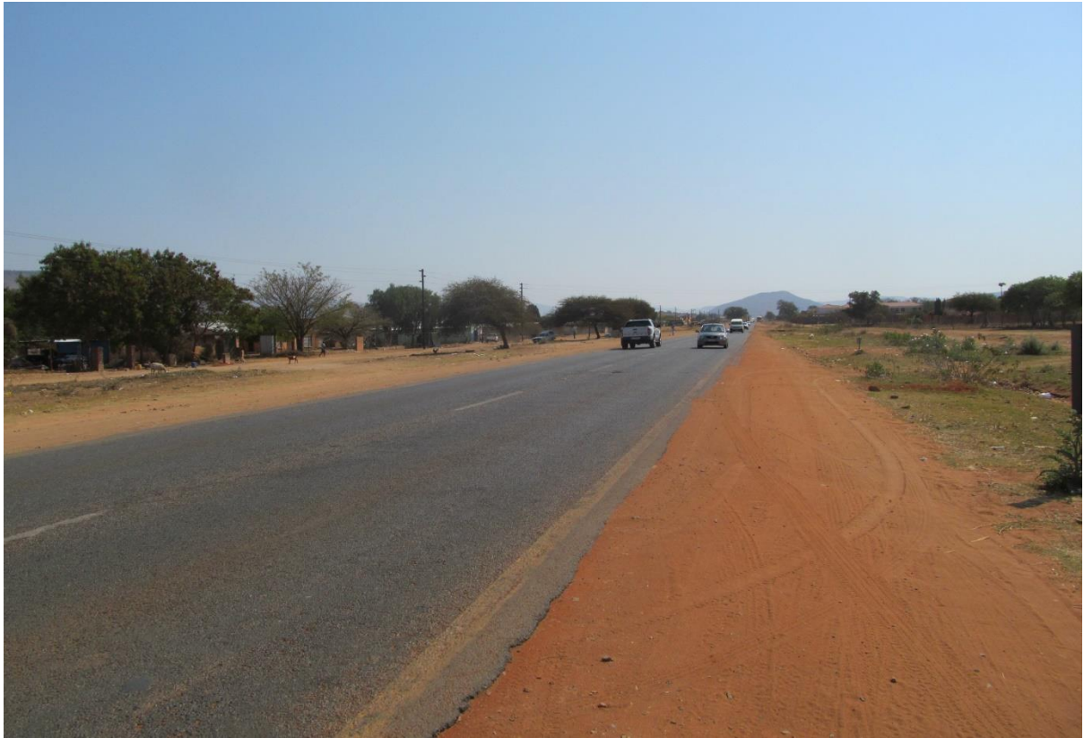
Photo 13: At km 137 to the North West
