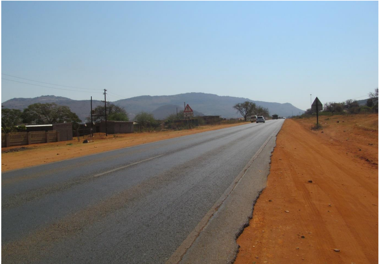
Photo 9: At km 127 to the North West
