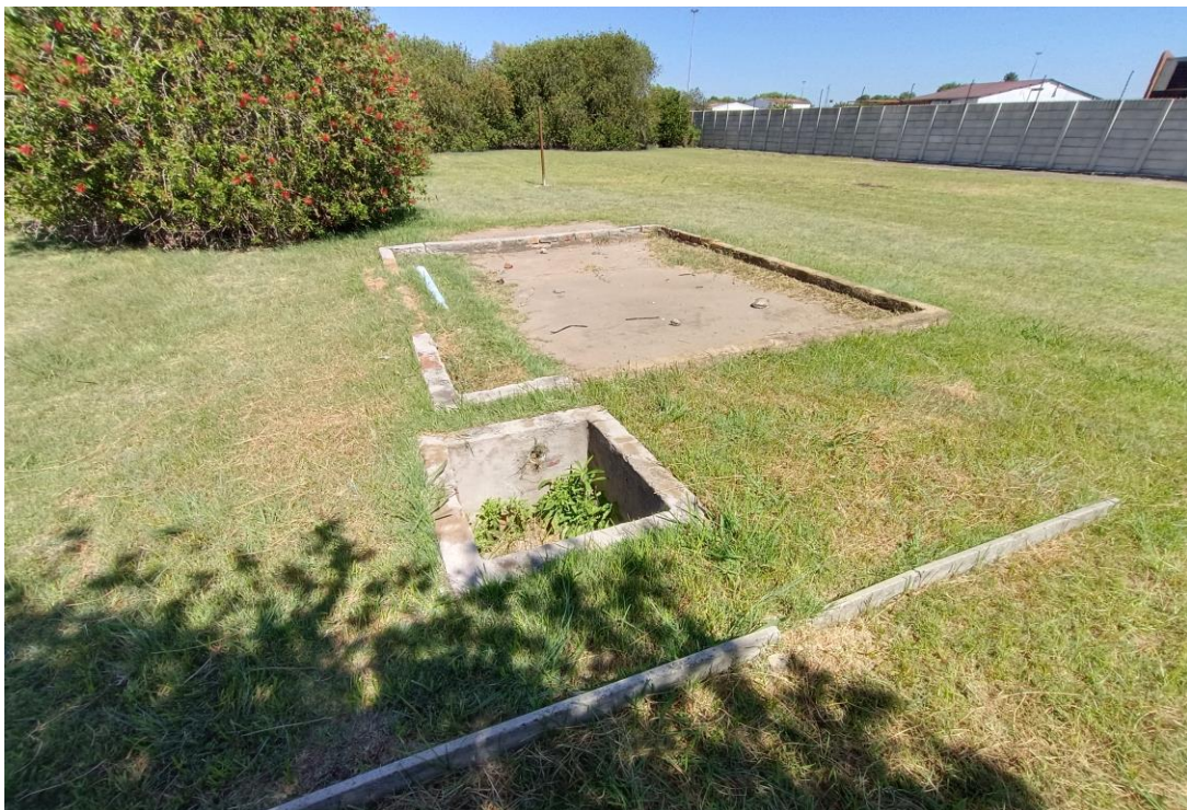
Figure 9: The remainder of a structure in the study & development area. These foundations are not of any heritage significance and likely less than 60 years of age (courtesy Eco Leges).
