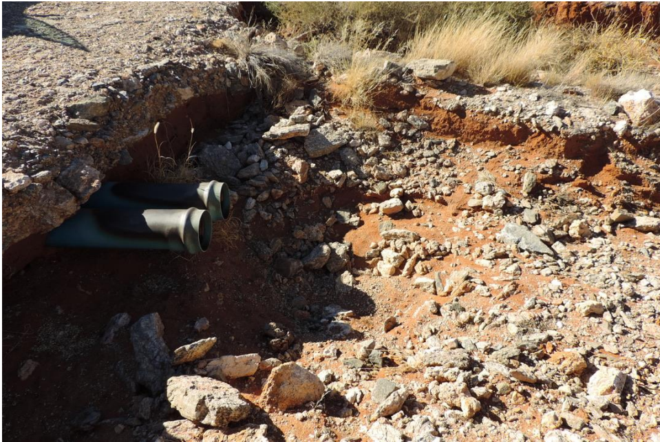
Figure 9 Old water flow infrastructure at a preferential flow path crossing along an existing farm road
