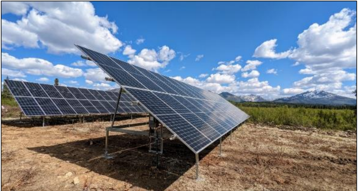
Figure 3: Photographic example of what the proposed PV could look like as single-axis tracker.
