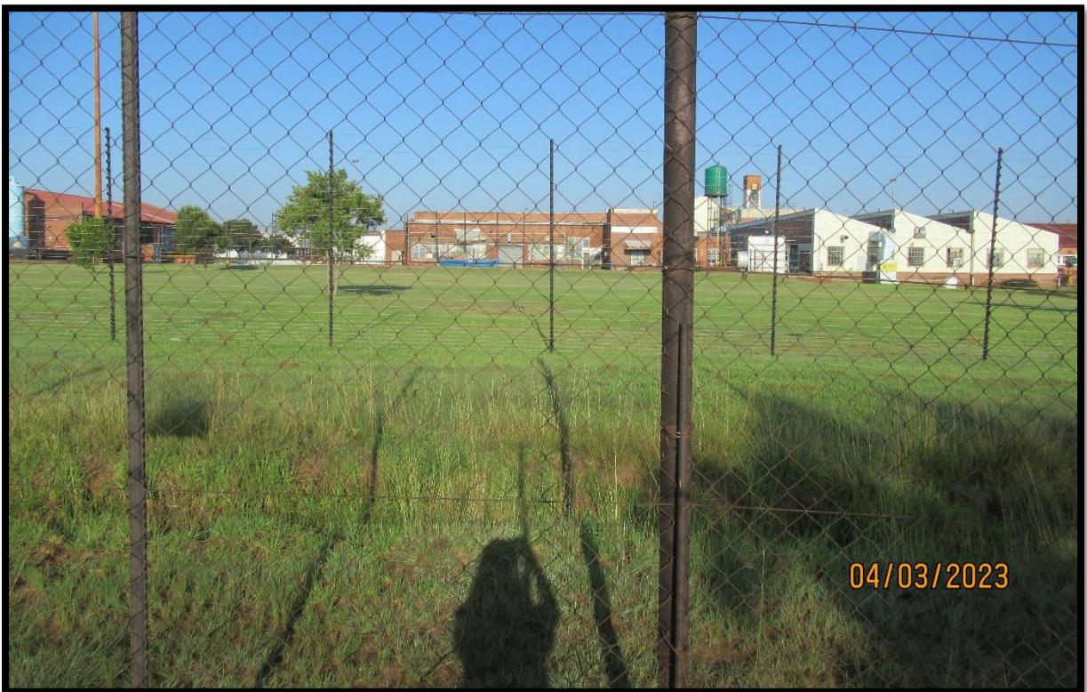
Figure 8: View in middle of project. This area will not be utilised.
