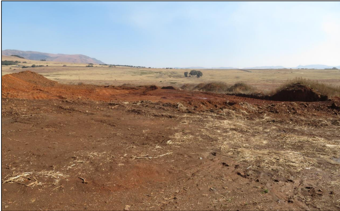
Plate 5-2: View of the shallow soils that are stripped above the mining front
