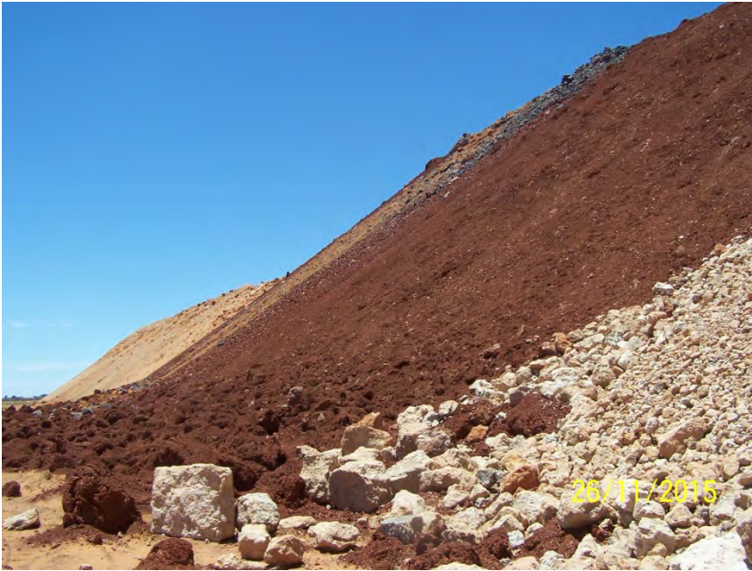
Figure B13: Side-slope of Northern dump with varying sections of calcrete (right), dark reddish clay (middle) and Kalahari sands (far left).
