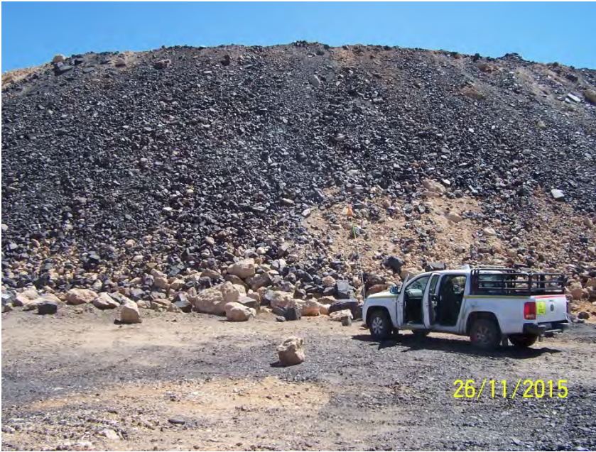
Figure B5: Side slopes of Western dump, mixture of shale and calcrete
