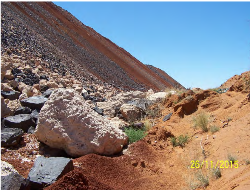
Figure B7: Side slopes of Western dump, dark reddish brown clay, shale and calcrete, partially mixed, and partially separated along slopes.
