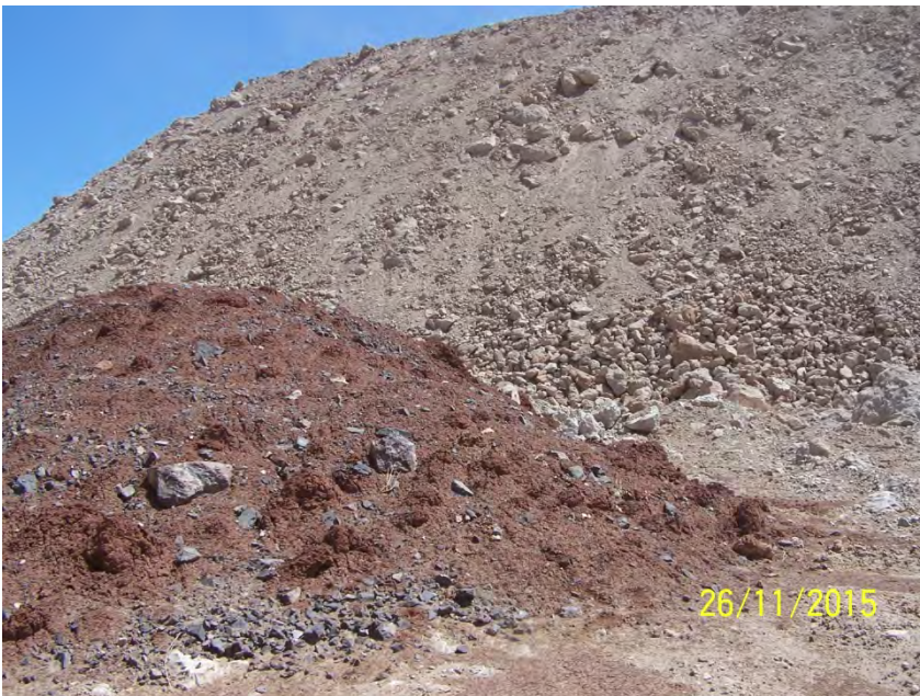
Figure B16: Base of Eastern dump, mostly calcrete side slope with reddish brown clay heap also mixed with shale at the base of the dump.
