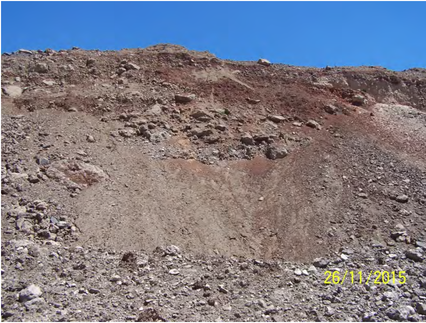
Figure 15: Side-slope of Eastern dump, portions conglomerate, portions calcrete, and portions reddish brown clay.
