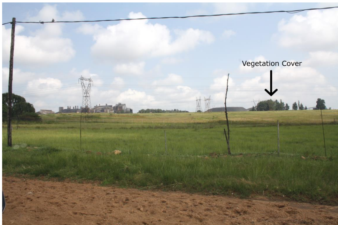
Figure 2: View from Clewer Agricultural Holdings (north) to the Transalloys Smelter Plant. (Note the potential effectiveness of planted vegetation cover in shielding the power plant structures).
