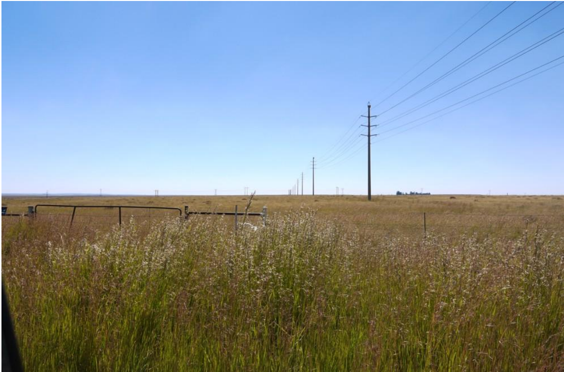
Plate 16 - A typical view along the line of a 132kV overhead power line with monopole towers.
