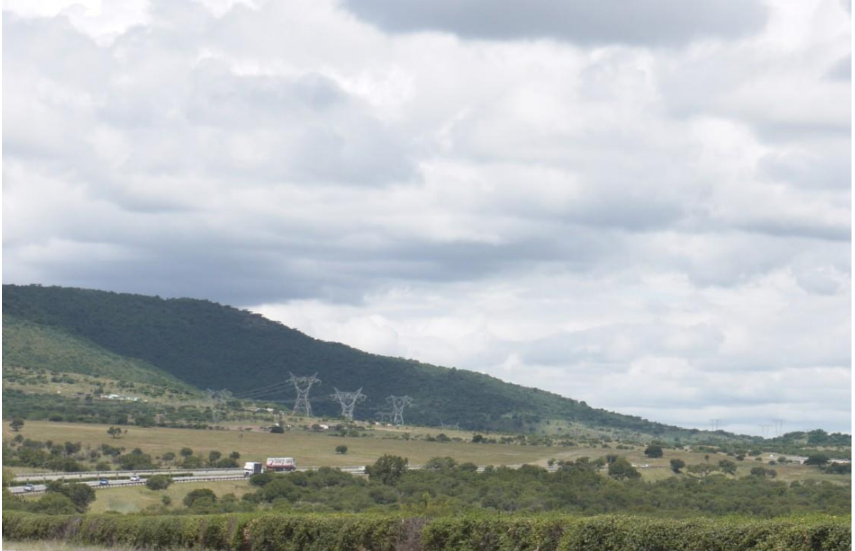
Plate 17 - 400kV double overhead transmission lines. Pylons are obvious in the mid distance (approximately 2-3km) but are not highly conspicuous at a distance (approximately 5-6km) as they cross the ridgeline.
