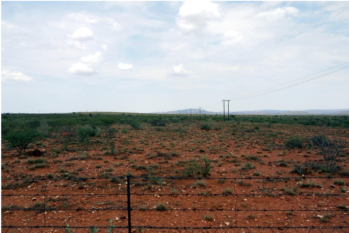
Plate 26, Existing overhead power line as seen from VP 3. Note: the proposed power line will follow this power line to the east of the N14 road crossing
