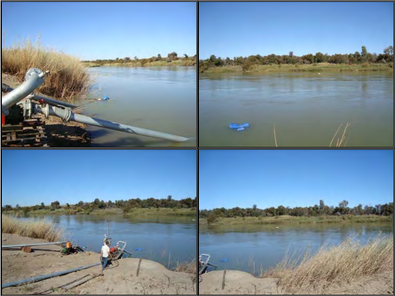
Figure 7: Various views of Site Bokpoort_1.
