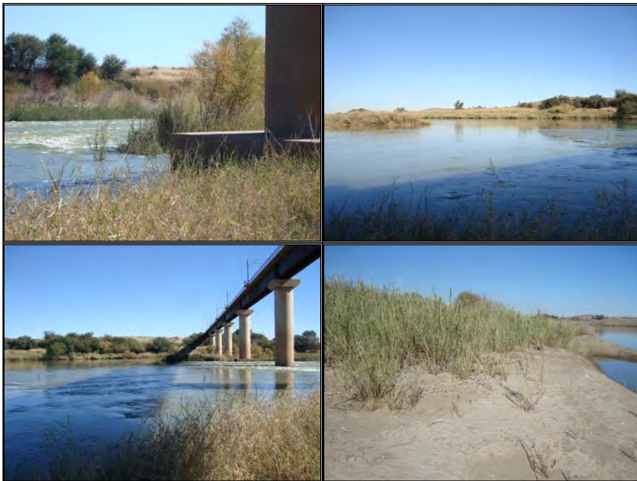
Figure 8: Various views of Site Bokpoort_2.
