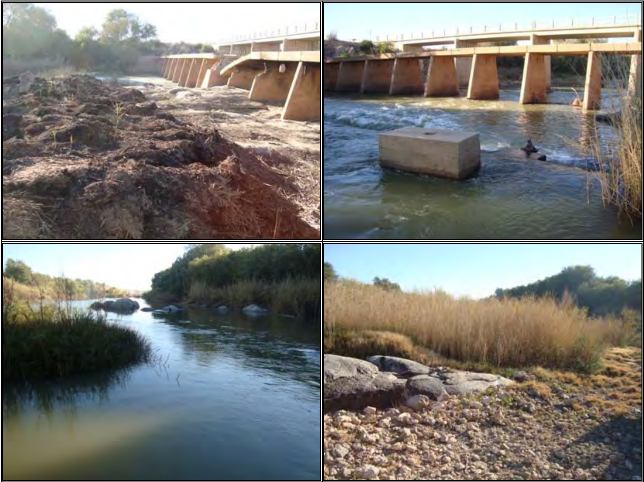
Figure 6: Various views of the site at Olyvenhoutsdrift.
