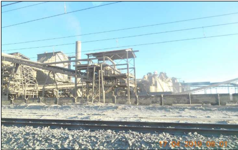
Figure 16: PPC Lime in Lime Acres, adjacent to Railway Line
