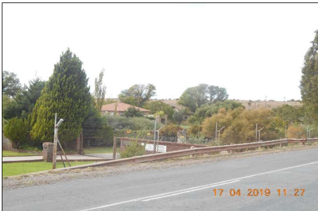
Figure 28: Affected Dwelling in Postmasburg (erected over the servitude)
