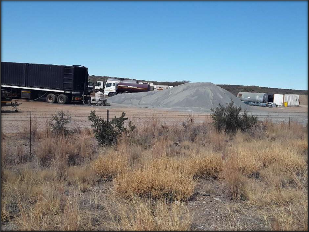
Figure 11: Roadworks next to the R31. GPS coordinates 28°19'05"S 24°12'49"E
