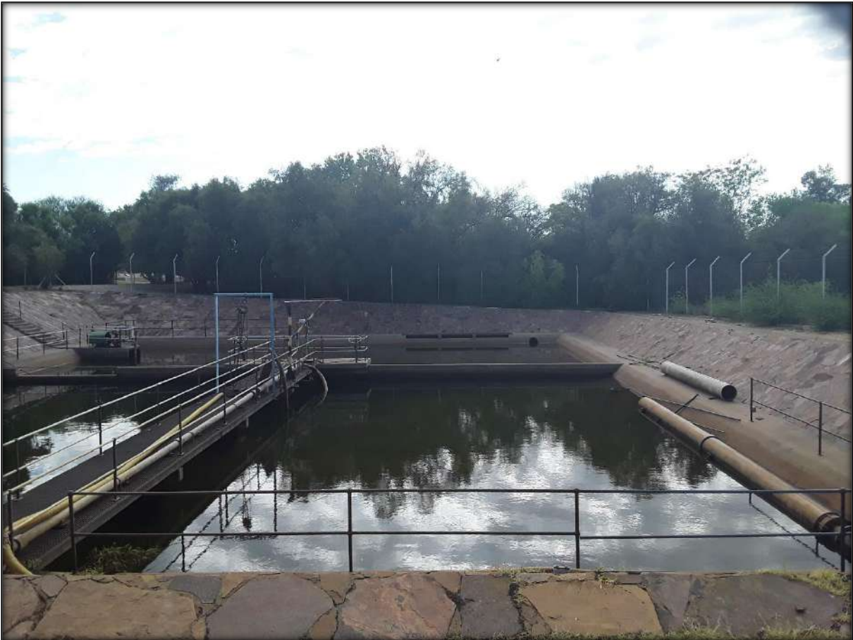
Figure 9: Start of the Vaal Gamagara Regional Water Supply Scheme: Phase 2 (VGRWSS-II) in Delportshoop
