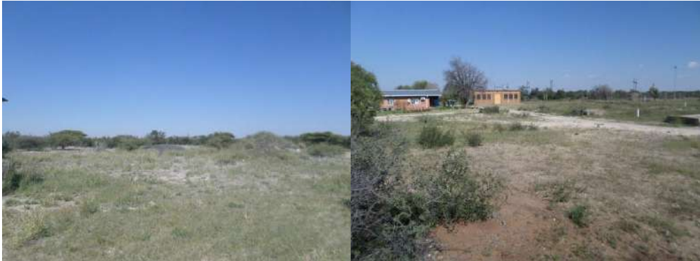
Figure 7: Kneukel Pump Station
