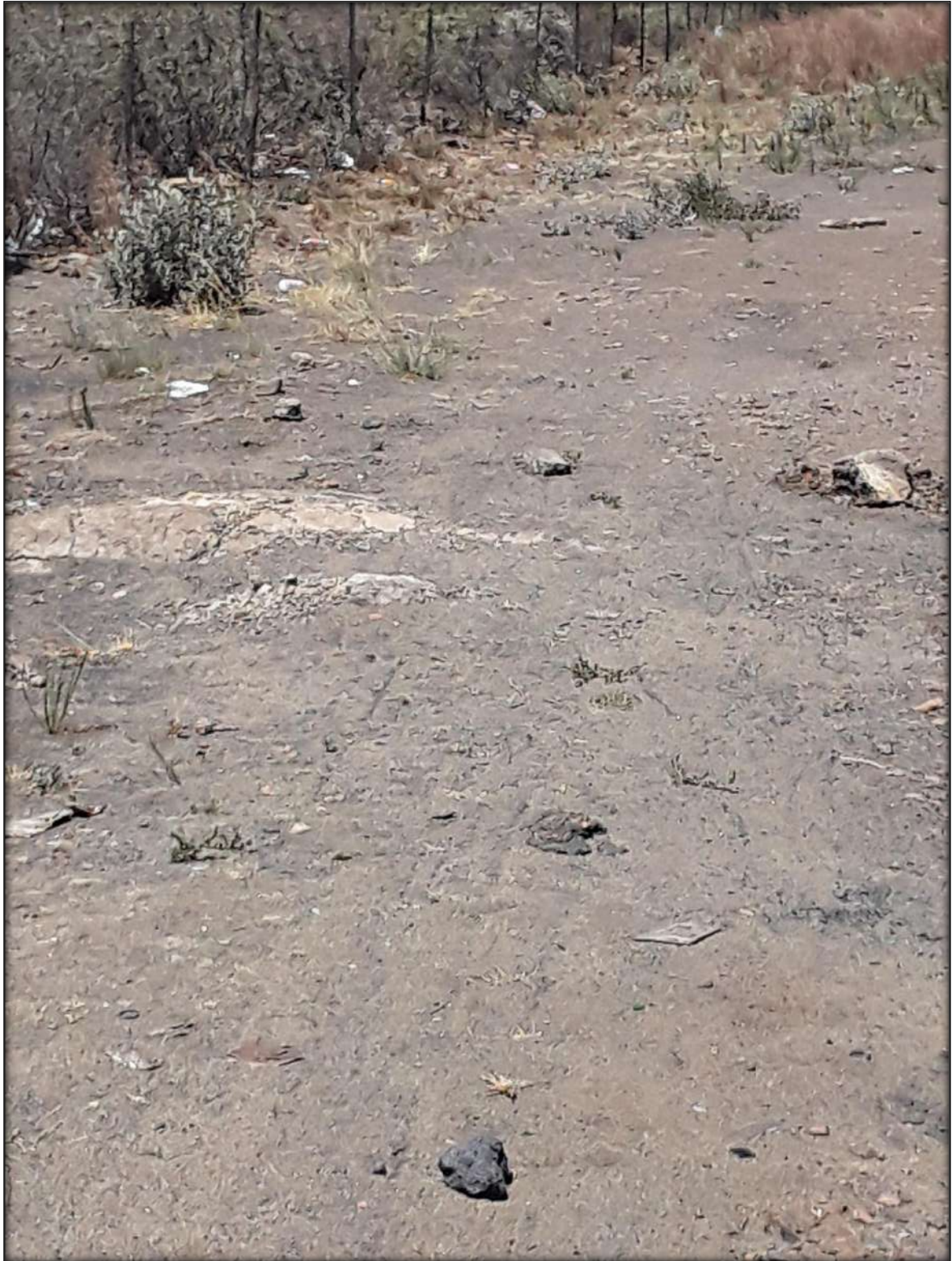
Figure 14: Roadside along R385. GPS coordinates 28°15' 57"S 23°32'48"E
