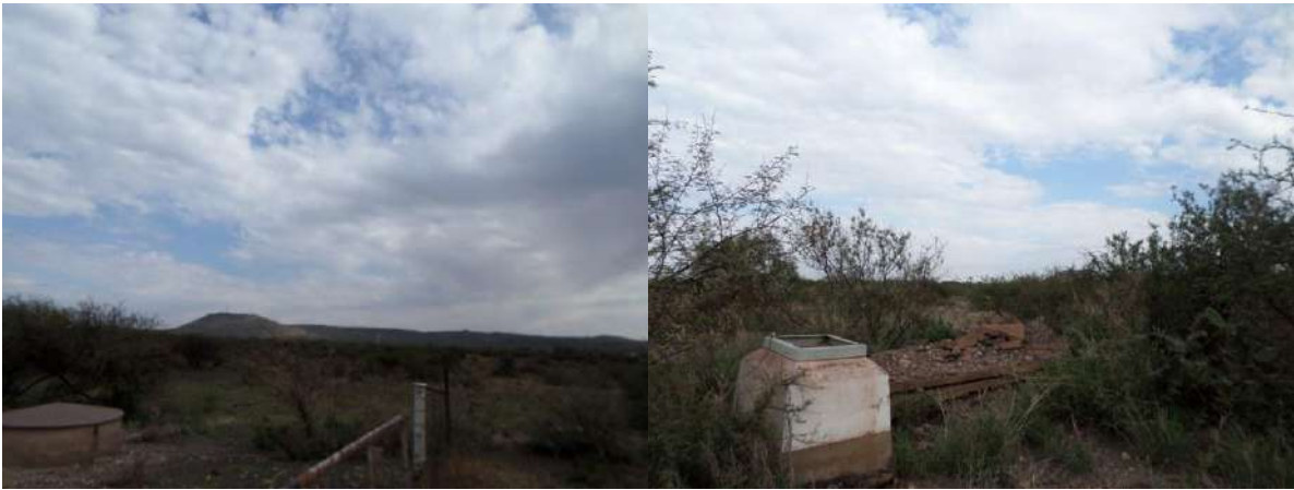
Figure 14: Old pipeline just near Boskop Farm and mine (en route to Olifantshoek)
