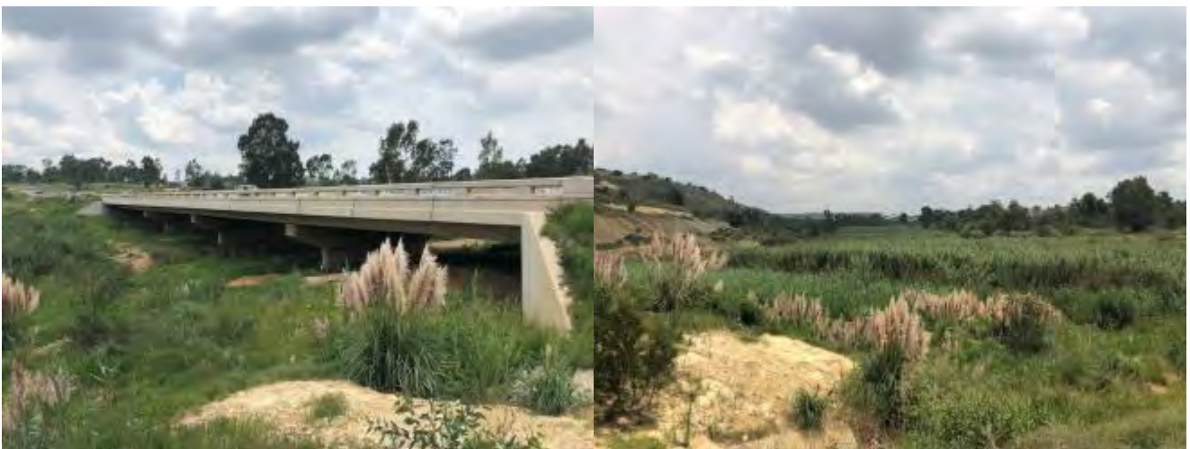
FIGURE 6-6: EASTERN STREAM - CULVERT 4
