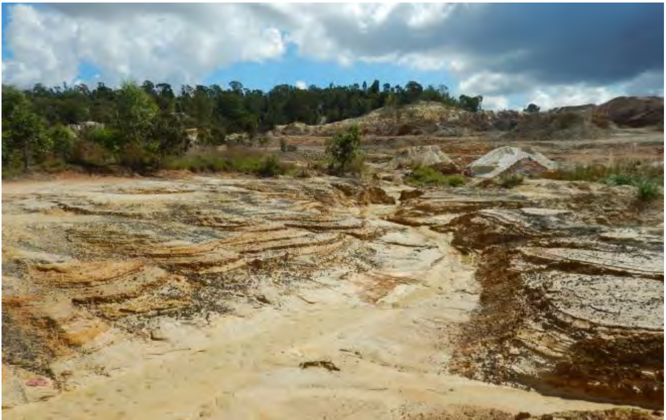
FIGURE 2-7: ERODED SLIMES MATERIAL FLOWING INTO THE NATURAL DRAINAGE CHANNEL (PHOTO: SLIMES EROSION)
