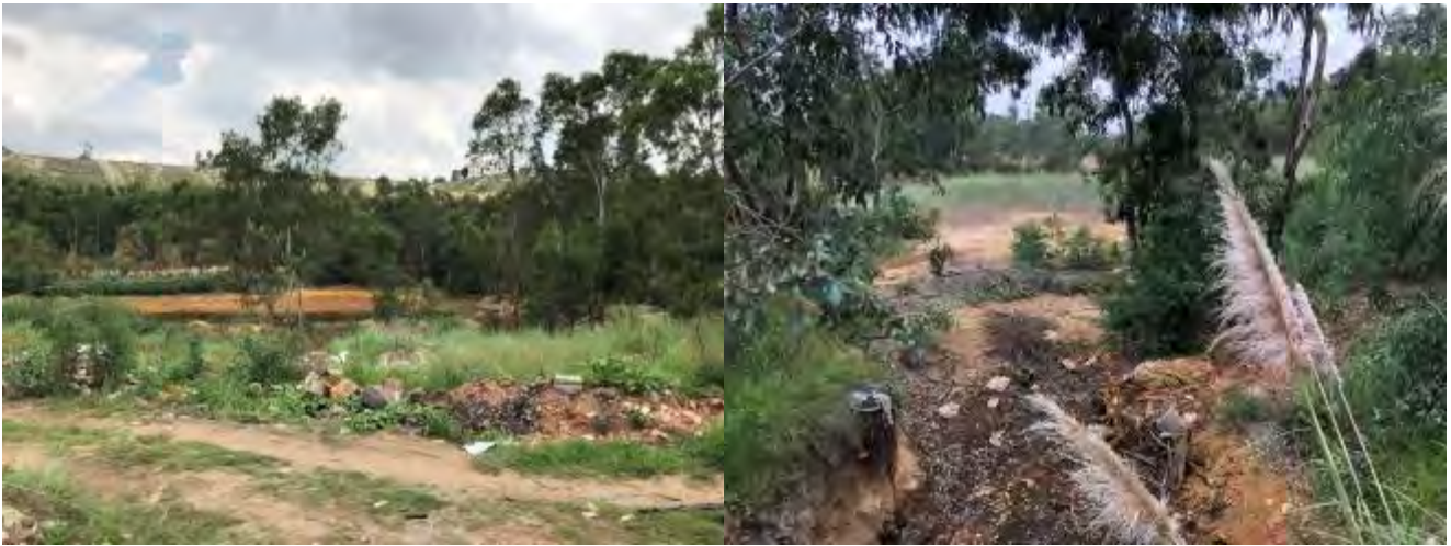
FIGURE 6-5: EASTERN STREAM - CULVERT 3
