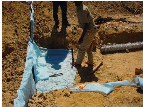
Figure 6: The photographs show the steps in the construction of a silt-screen. Girls from two schools in Pretoria on the Mabula Game farm carried out this exercise. In photo 1 the trench is dug across the erosion channel and Y standards are placed to form the main part of the structure. In photo 2 the Y standards are connected with stay wires and covered with wire mesh. The structure is then covered with a biodegradable geo-textile in photo 3. In photo 4 the structure is completed by adding an apron, made of geo-textile and wire mesh.
