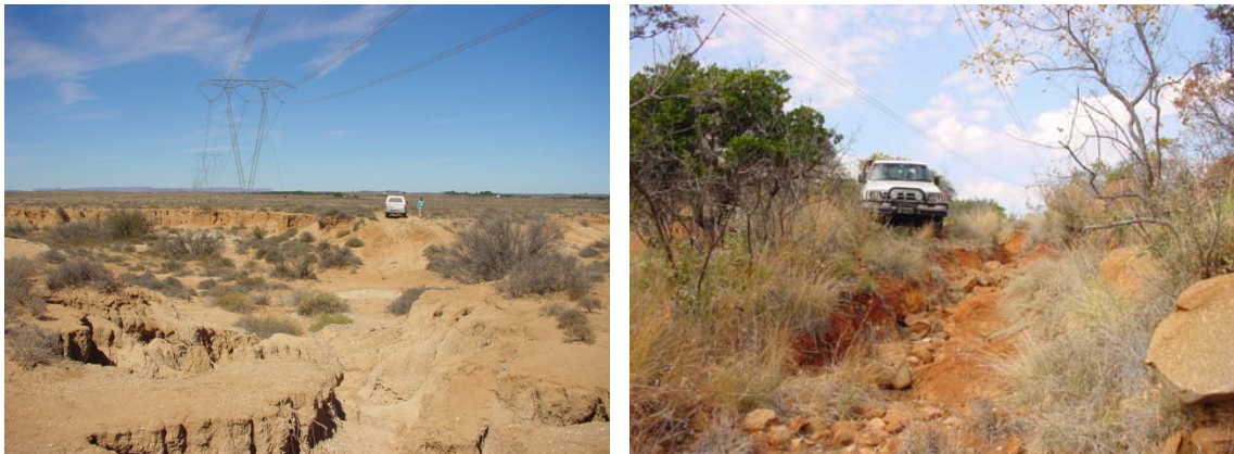
Figure 2. Examples of erosion in the servitude, which hampers access during maintenance and emergencies.
