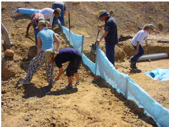
Figure 6: The photographs show the steps in the construction of a silt-screen. Girls from two schools in Pretoria on the Mabula Game farm carried out this exercise. In photo 1 the trench is dug across the erosion channel and Y standards are placed to form the main part of the structure. In photo 2 the Y standards are connected with stay wires and covered with wire mesh. The structure is then covered with a biodegradable geo-textile in photo 3. In photo 4 the structure is completed by adding an apron, made of geo-textile and wire mesh.
