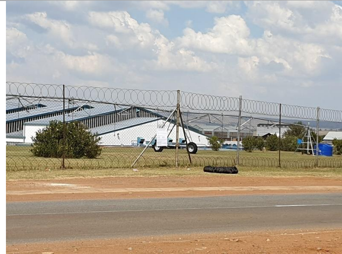
Business and fencing along pipeline route which is a common land use within the area
