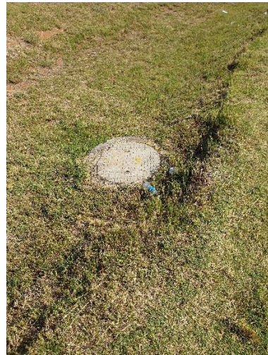
Maintenance hole for existing buried pipeline within the development corridor
