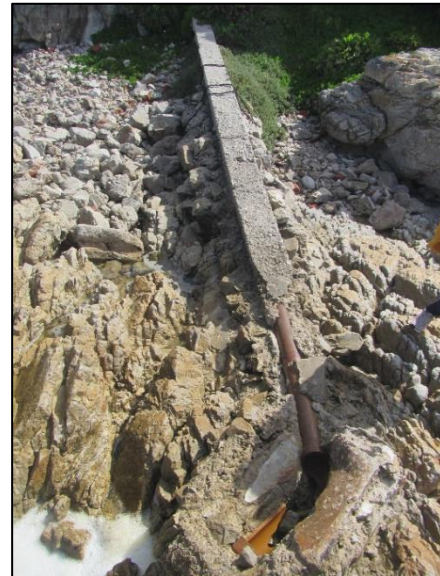
Remnants of old pipeline on the rocks below the old Bay View Hotel site. Several examples were seen, largely in disuse.
