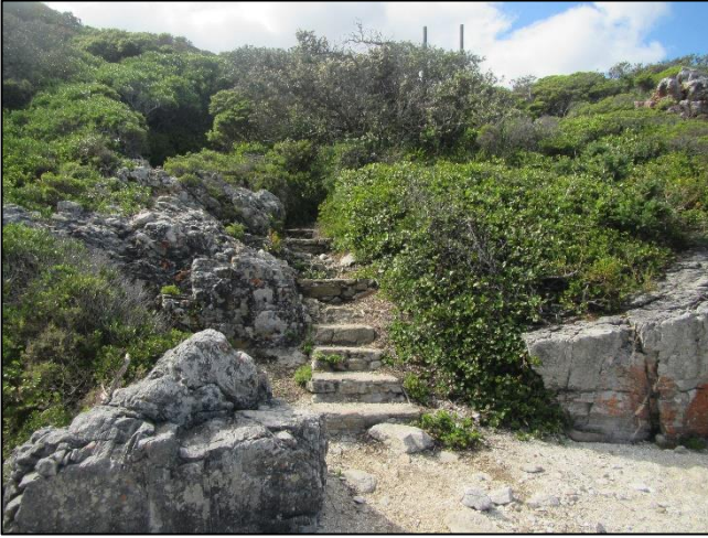
Part of the old walkway with steps made of stones and cement. This is just before the section where the new path would begin. This part may be upgraded as part of the new project but the path would not be widened.
