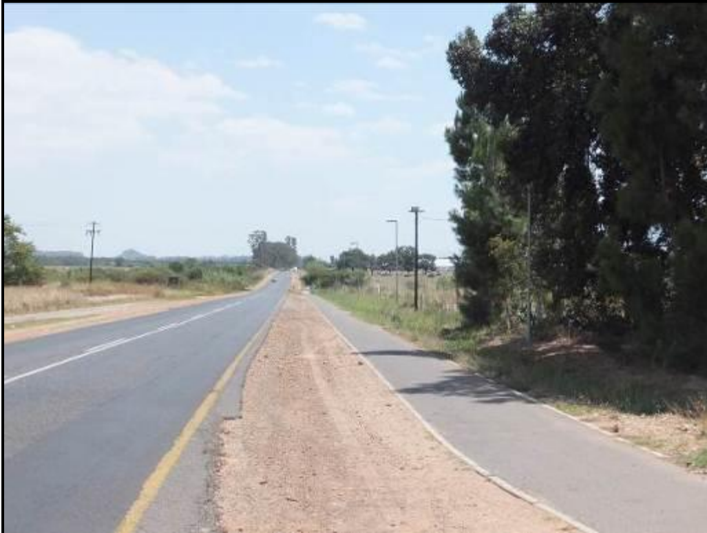
Photograph 1.8: Pedestrian pathway adjacent to R 45
