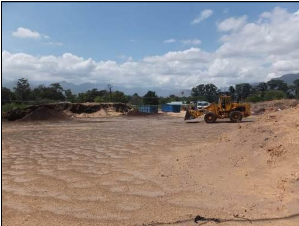
Photograph 1.14: Wood processing operations on the site
