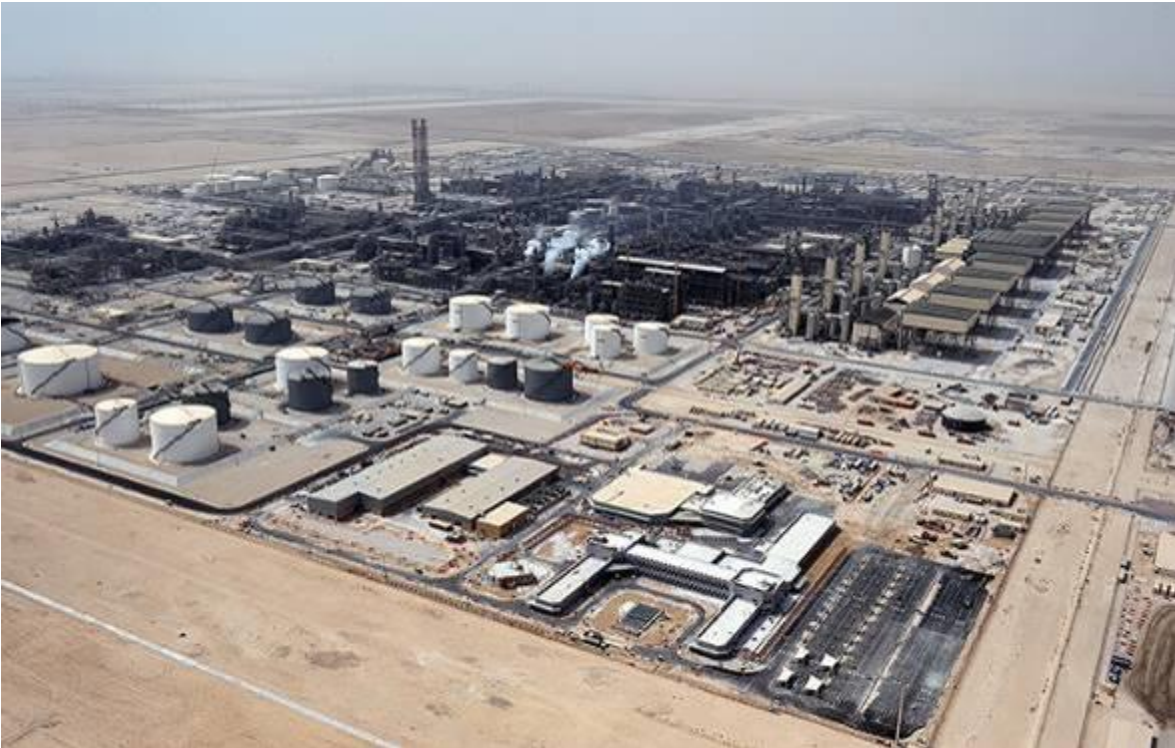
Photograph 3.1: Secunda Sasol Facility
