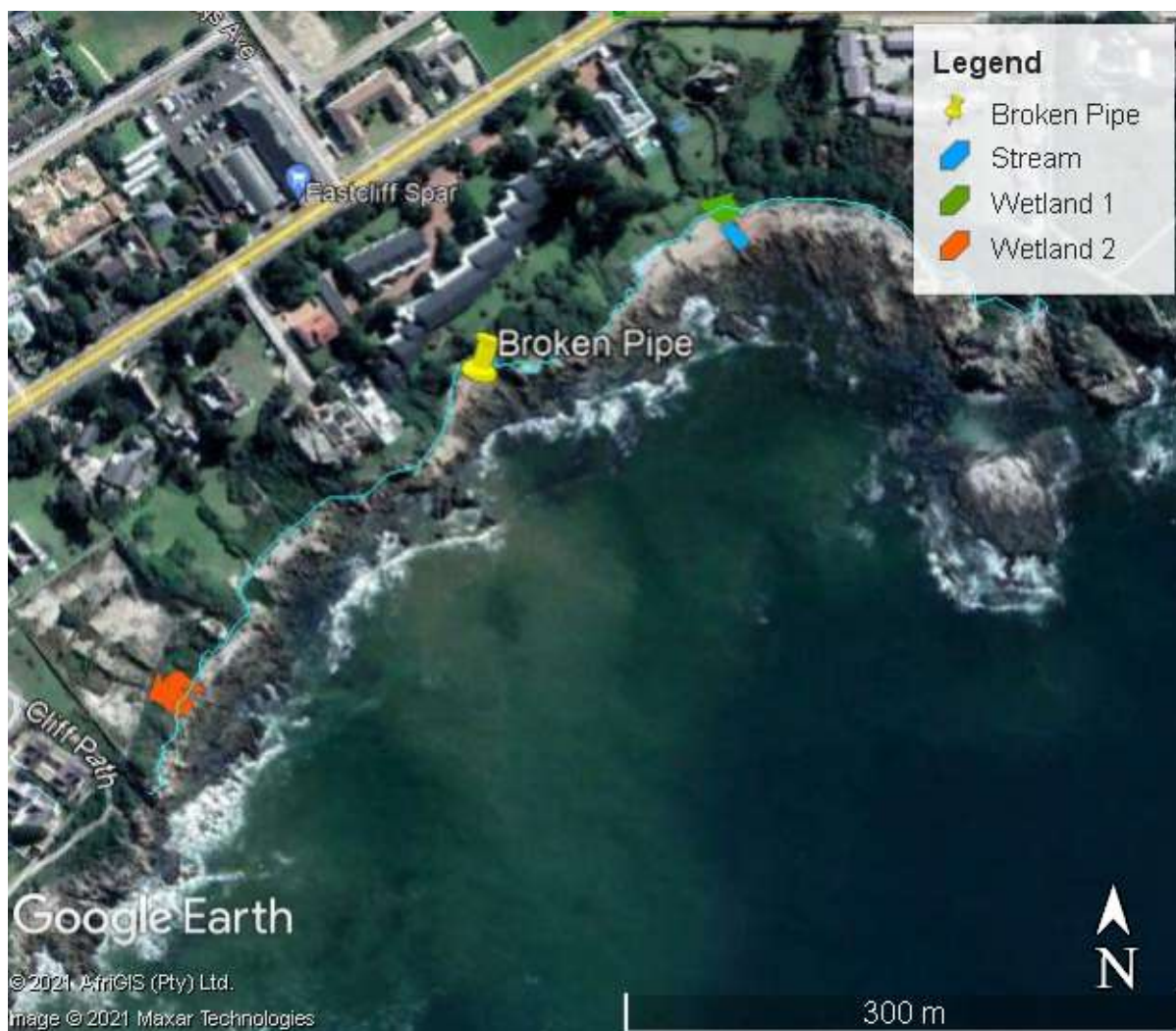
Figure 10: Location of the two delineated wetlands, stream and the broken pipe in relation to the high-water mark (shown as a light blue line).
