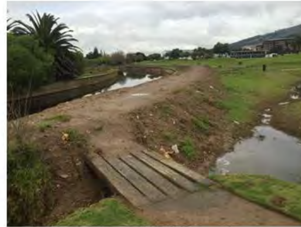
Photo N Creation of berms along the eastern channel of the Liesbeek River, to reduce flooding
