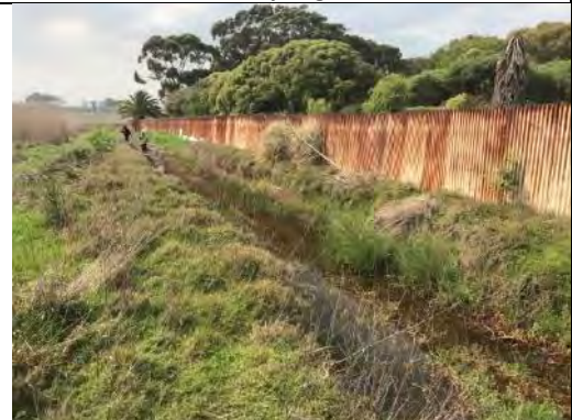
Photo X Trench along the “fenced” edge of the SAAO – purpose of trench assumed to be to convey water from the SAAO boundary to deep water habitats to the south
