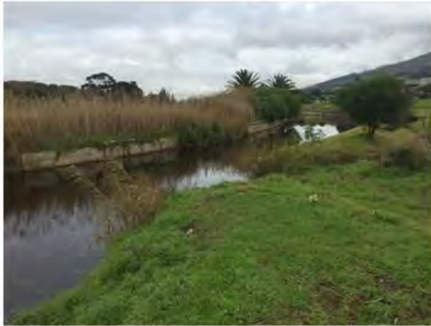
Photo M Canalised section of the eastern channel of the Liesbeek River
