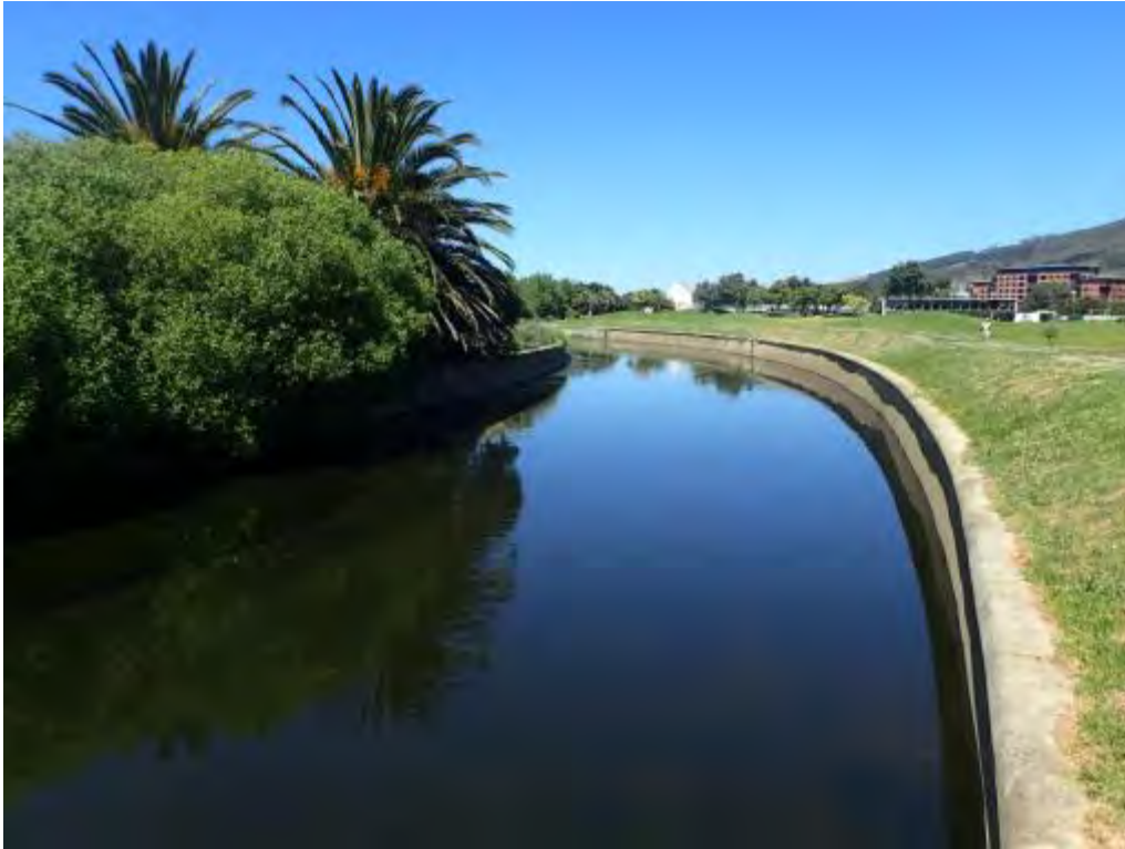
Plate 21. Canalised section of Liesbeek River, forming the eastern boundary of the River Club site. Canalisation offers very little rehabilitation potential for the river
