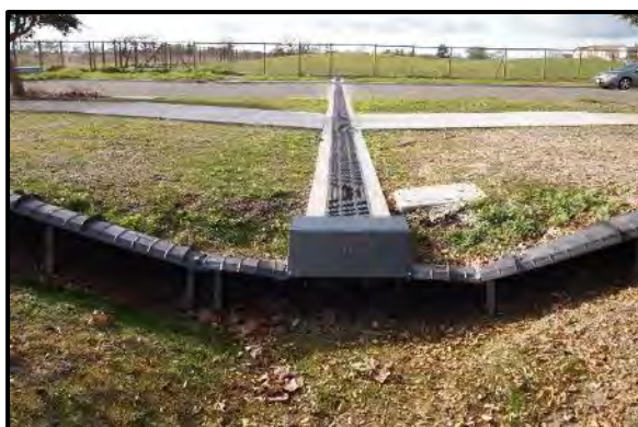
Figure 25: Underpass with a grid roof, designed for toads and other small faunal species.
