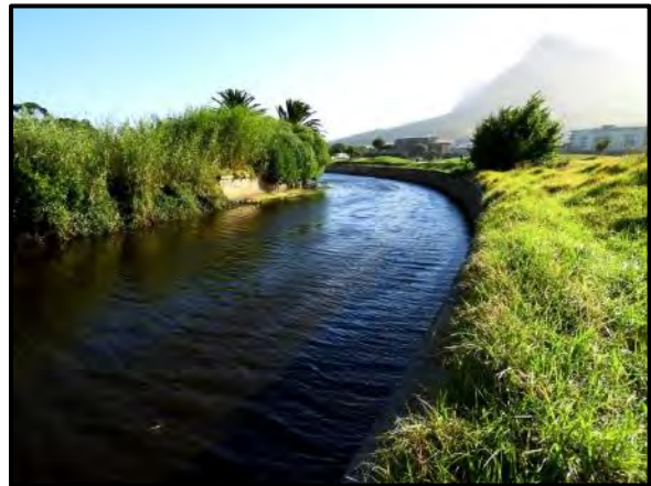
Figure 4: A canalised portion of the Liesbeek River that flows along the eastern boundary of the River Club property.
