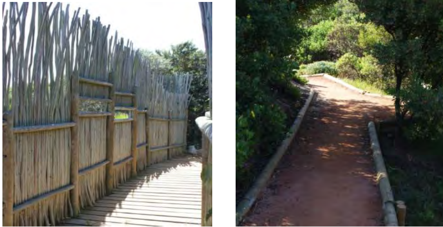
Figs. 16 & 17: Examples of a) an inexpensive screen that enables viewing of wildlife with minimal risk of disturbance; and b) a wheelchair suitable walking trail through bush habitat. Note the passing bay and the sense of exploration created by the effect of the trail winding out of sight. Both these sorts of features would be appropriate for the outer, relaxed, trail in the apron.
