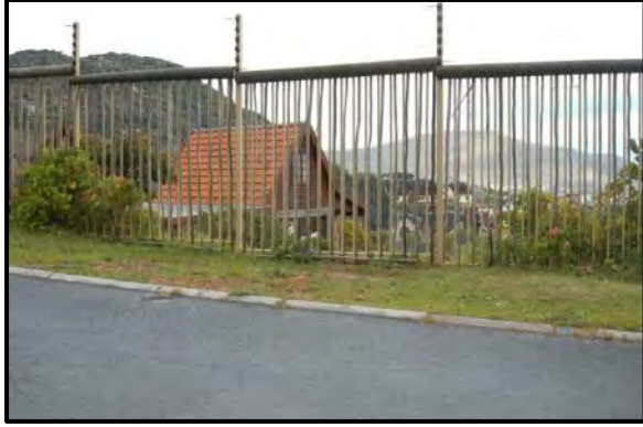
Figure 27: An example of permeable toad-friendly fencing in a residential setting.
