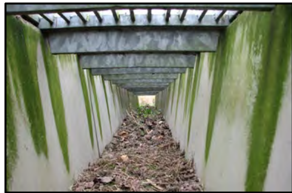
Figure 24: Underpass with a grid roof.
