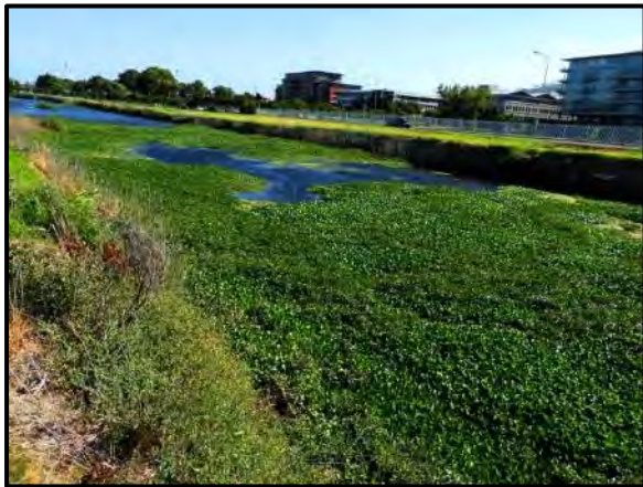
Figure 3: The historic unlined reaches of the Liesbeek River, along western and north-western boundary of the study area.
