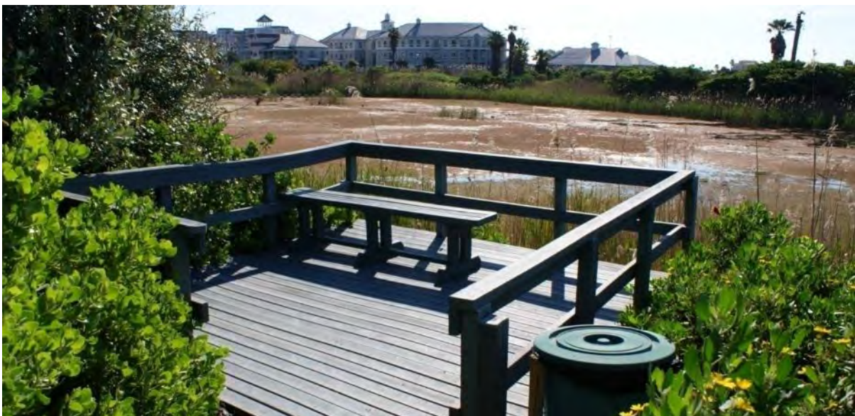
Fig. 15. A public viewing unit – constructed with “plastic wood”. Not all viewing areas need be so fancy though decking is important in wet situations where heavy treading would soon result in a muddy mess.
