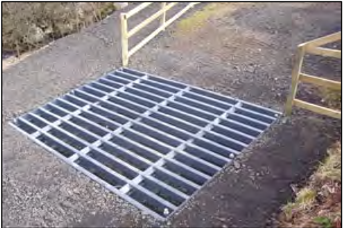
Figure 29: An example of a cattle-grid structure that can be used strategically to prevent toads from entering specific hazardous areas, and to redirect them by means of tunnels to safe terrain.
