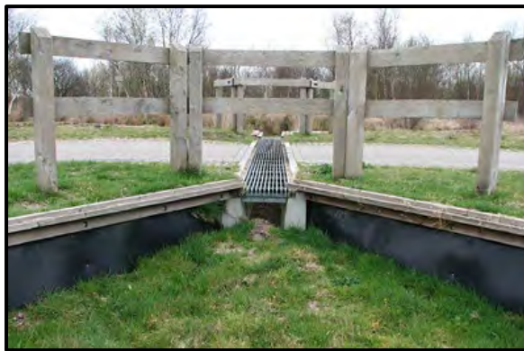
Figure 23: Underpass with a grid roof and directing walls.
