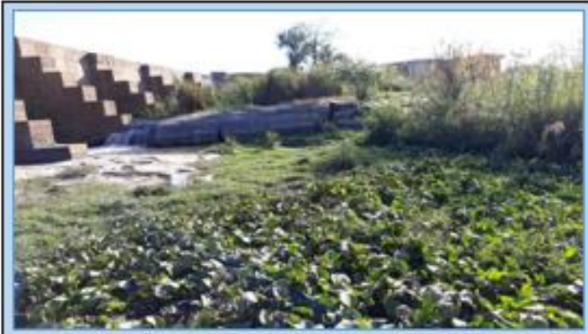
Plate 1: Upstream view of H-US-KF (2018-05)
