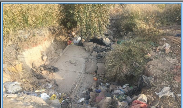
Plate 21: Downstream view of KGT (2019-06)
