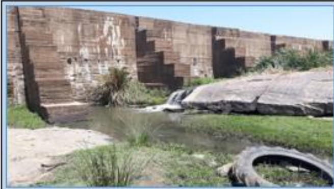
Plate 3: Upstream view of H-US-KF (2018-10)
