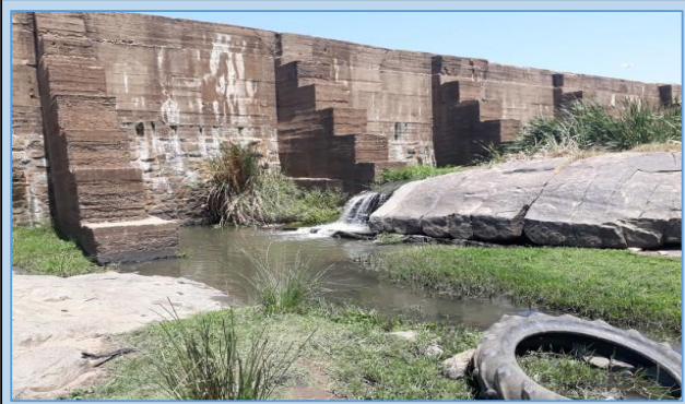
Plate 3: Upstream view of H-US-KF (2018-10)
