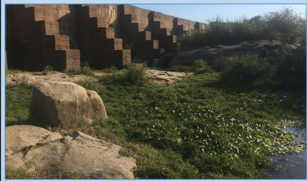
Plate 1: Upstream view of H-US-KF (2019-06)
