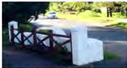
Fig. 34 Culvert crossing and footbridge (Briel, 2015)
