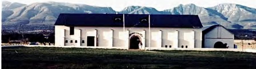
Fig. 112 Market building example Martin Kruger Architects - Birkenhead Brewery.
