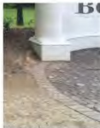
Fig. 43 Example of exposed aggregate, brick and local stone as road surfaces at Boschendal (Briel, 2015)
