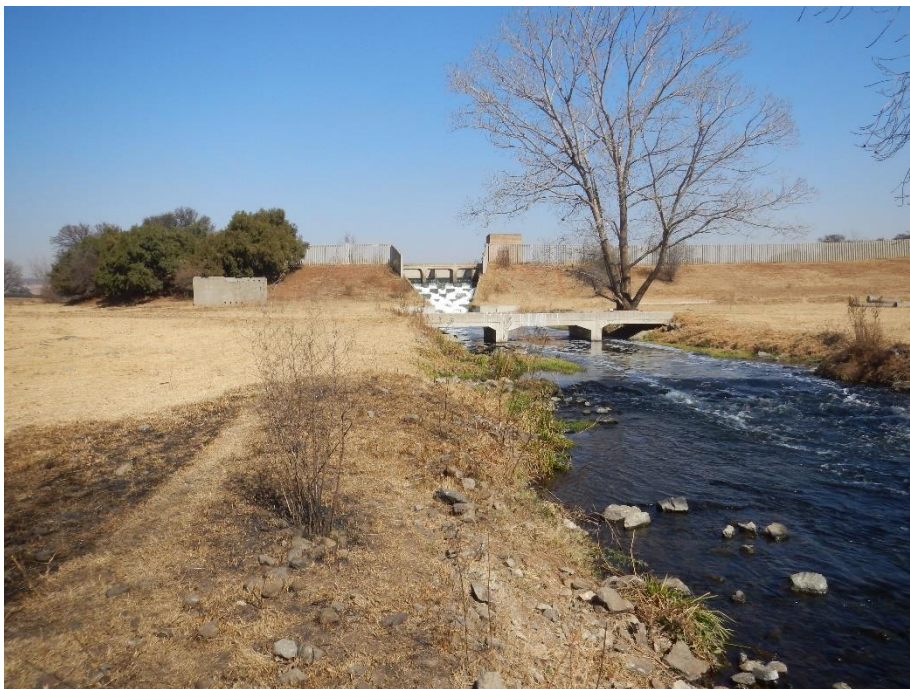
FIGURE 8: OUTLET FROM THE OXIDATION PONDS INTO THE MAIN CHANNEL
