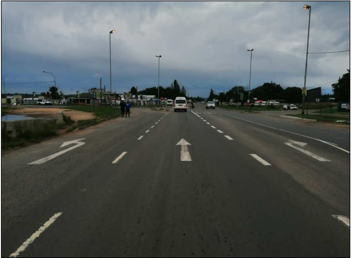
Figure 4.1: Springs Road / Pretoria Road (M44) Junction
