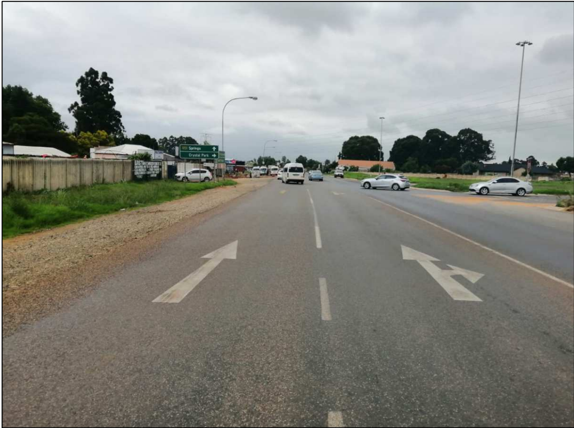
Figure 4.3: Springs Road / Kingsway Road / Durandt Road / Kerk Street Junction
