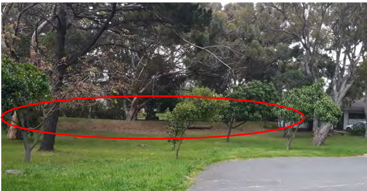
Figure 2-6 Berm on the South African Astronomical Observatory (SAAO) side of the Liesbeek Canal – constructed sometime between 2013 – 2015
