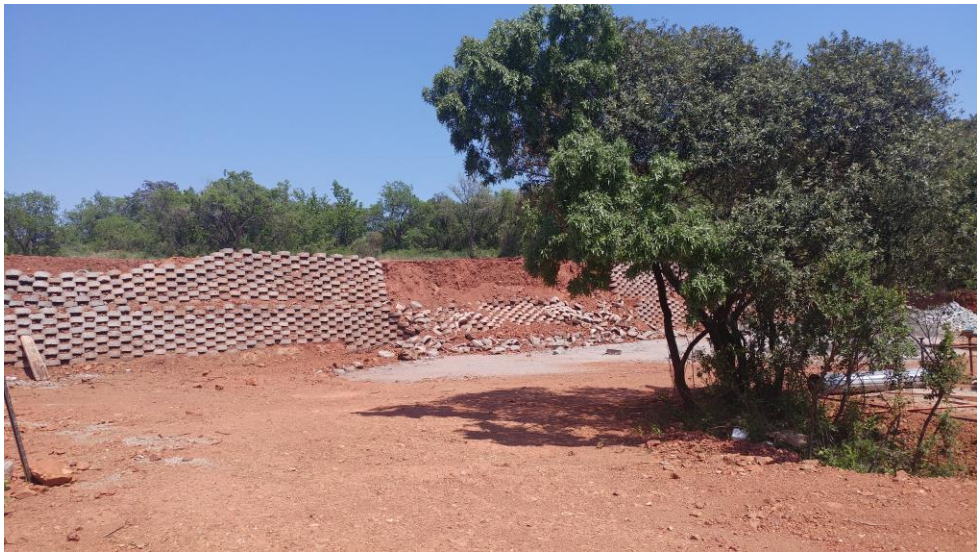
Figure 7: Site 1 – note the openness and concrete being constructed to prevent erosion.
