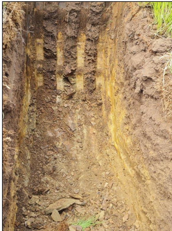
Fig. 5: General view of test pit 5
