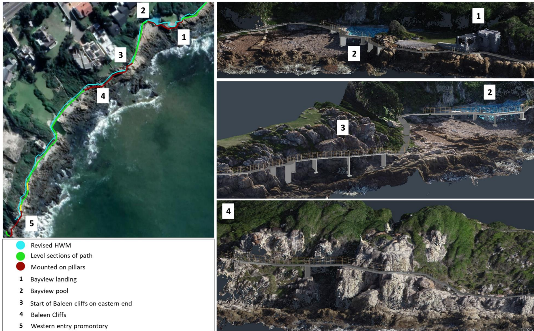
Figure 12 In some sections, the cliffs and therefore the proposed path, extend into the intertidal zone. For this reason, the proposed path will be raised and mounted either against the cliff wall or on pillars. These elevated sections will occur at the (1) Bayview landing; (2) Bayview pool; (3&4) Baleen cliffs; and (5) Western Entry Promontory.
