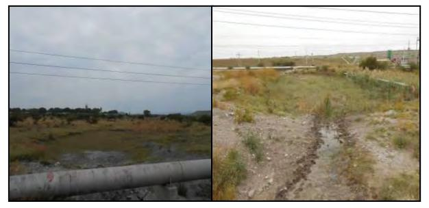
Figure 19: Erosion observed along the pipeline crossing within Klipgatspruit.
