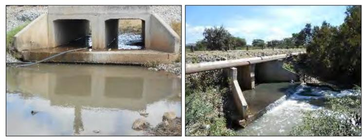
Figure 71: Culvert Bridge indicating elevation drops at biomonitoring sites.
