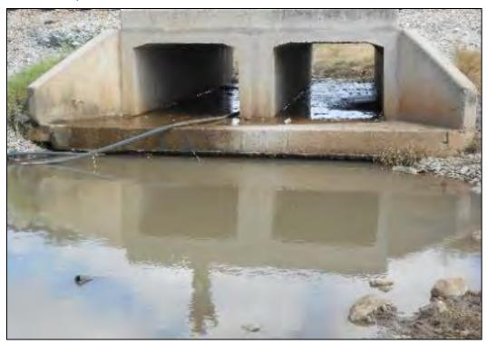
Figure 69: Culvert Bridge indicating the scouring and undermining of the Culvert structure resulting in altered stream hydrology.
