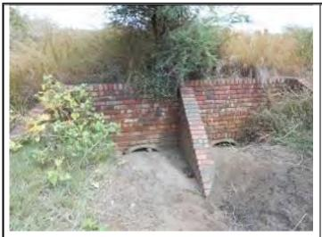
Figure 58: Upstream view of the SASS 35A site located on the Wildebeesfonteinspruit. The site was dry at the time of the assessment and culverts largely silted up.
