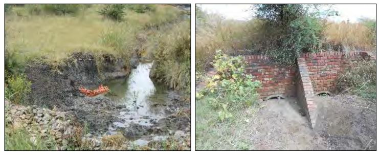
Figure 68: Erosion and Sedimentation evident at crossings within the RPM boundary.
