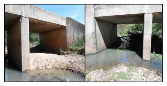
Figure 16: Sediment deposition and debris within the stream.
