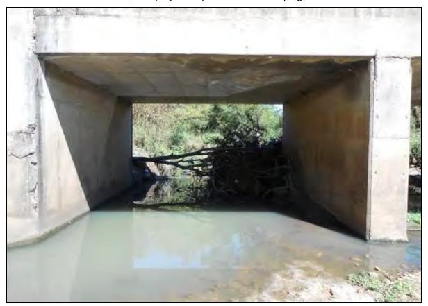
Figure 70: Blockages present at monitoring sites, restricting movement of debris downstream.
