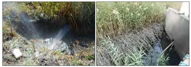
Figure 73: Leaking pipes within the RPM operations boundary.
