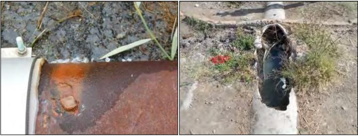
Figure 74: Leaking pipes within the RPM operations boundary and broken pipes within the rural residential area.
