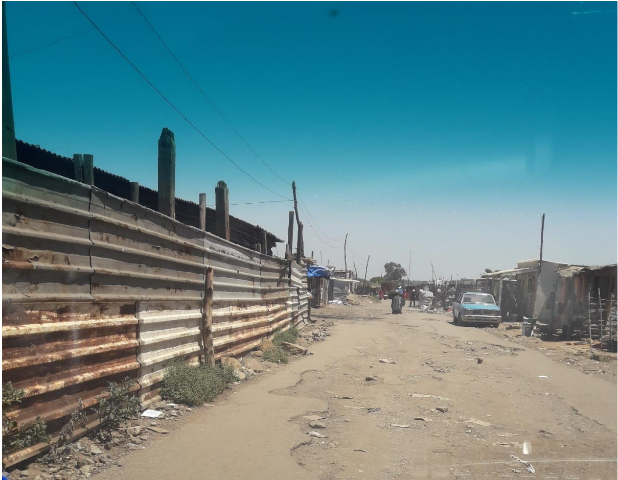
Figure 5: Station Road looking southwards, close to the intersection with the R29 (Main Reef Road). Both sides of the road are lined with informal structures and it was not possible (or safe) to access the land to the west (right of the photo). Note that the original tarmac of the road surface is mostly missing.
