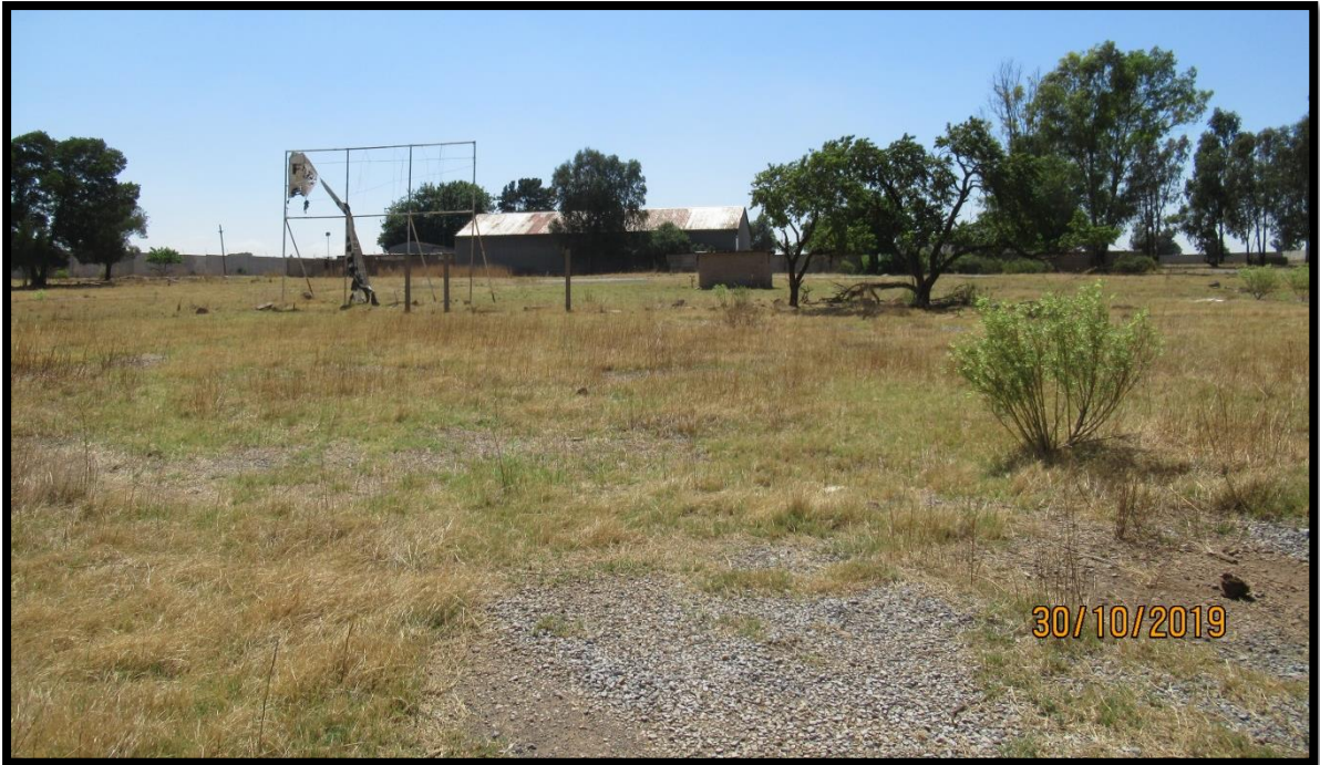
Figure 7: View towards gate and site office.
