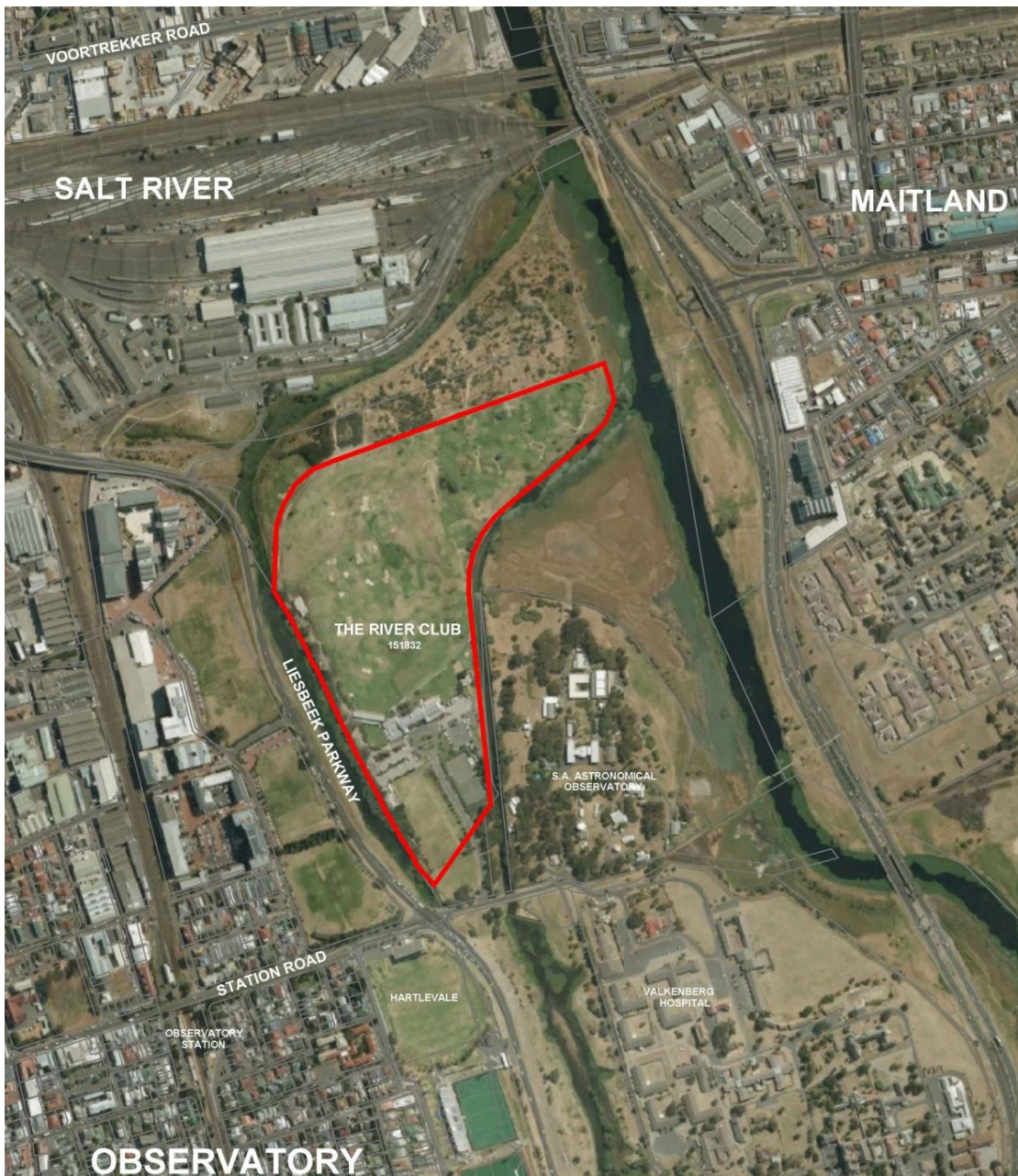
Figure 23. The River Club site as at present: The “existing rights” or “no-go” alternative.
