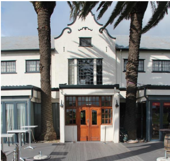
Illustration 7: Entrance to the River Club building from the north-east (SST, #11, July 2019)
