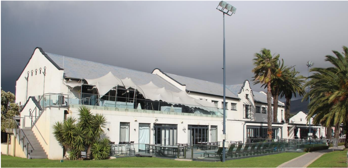
Illustration 6: The main River Club building from the north-east (SST, #11, July 2019)
