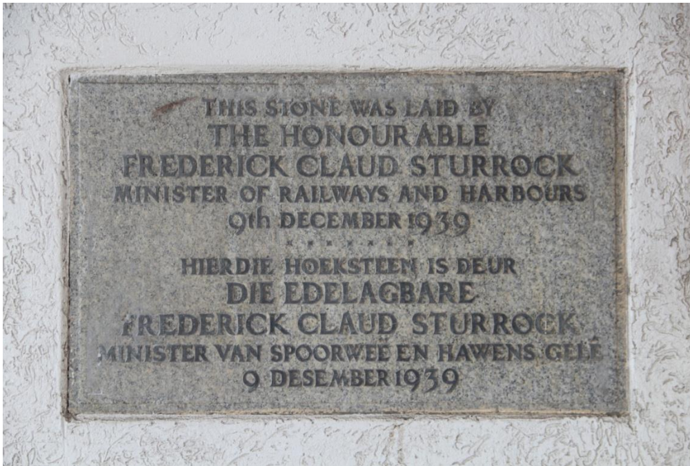
Illustration 3: The 1939 foundation stone (SST, #22, July 2019)
