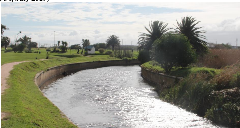
Illustration 15: View north up the canalised Liesbeek River; River club site to the left and the SAAO site to the right (SST, #10 July 2019)
