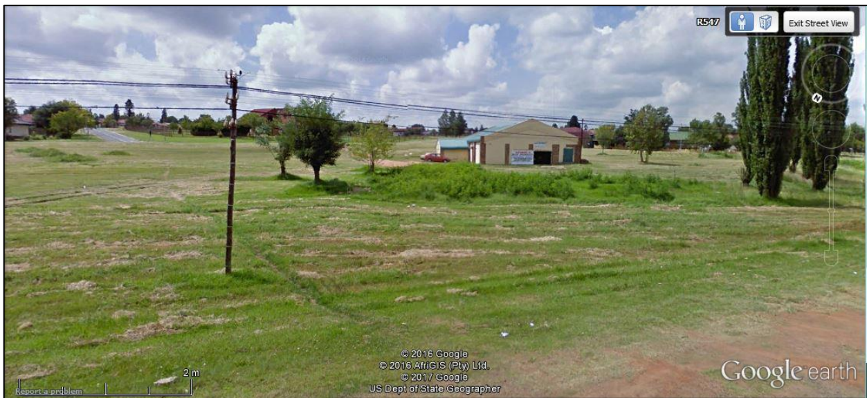
Figure 7: View of the site facing towards the southeast from the R547. Source: Google Earth Street View. Image dated February 2010.
