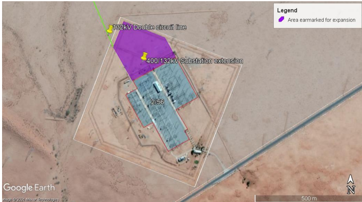
Figure 3-6: Area earmarked for the expansion of the Aggeneis substation
