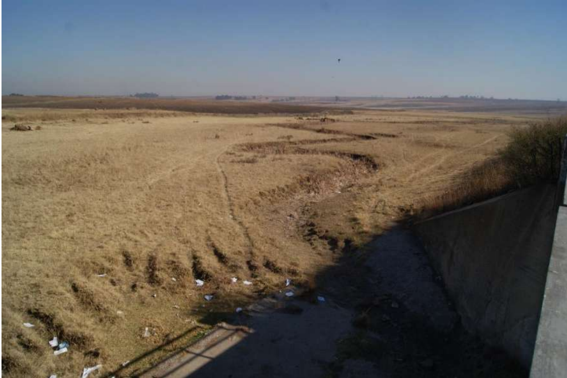
Upstream culvert along R544 (26° 13'56.5" S 29° 19'47.4" E)
