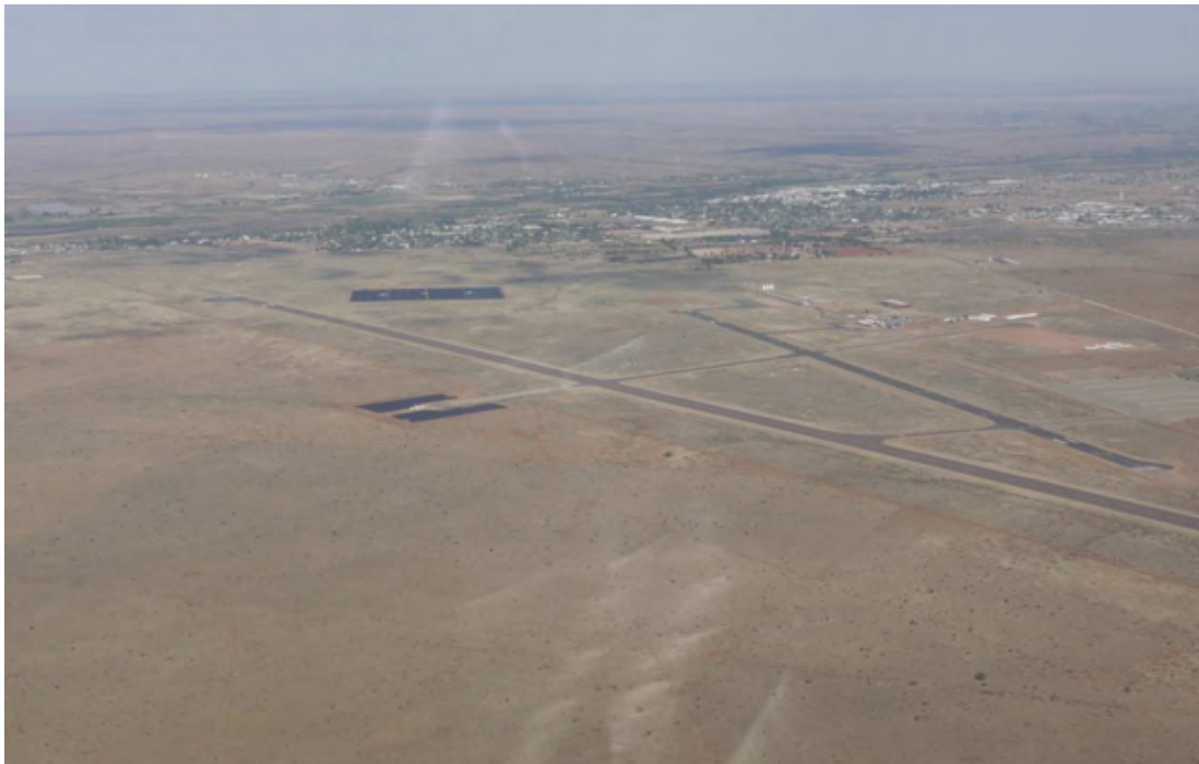
Plate 21 , Existing Solar Arrays at Uppington Airport as seen from the air
