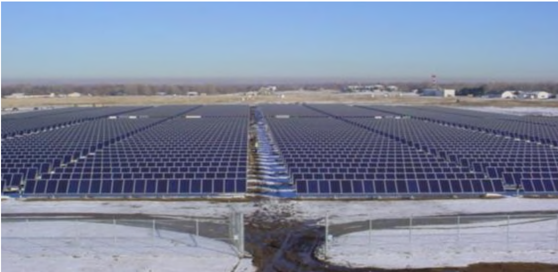
Plate 18, PV array viewed from above. Note the array rows are read as one and have a similar impact as the roof of a large industrial building might.
